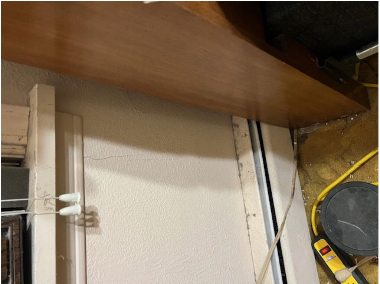
Signs of foundation crack on north bedroom wall
