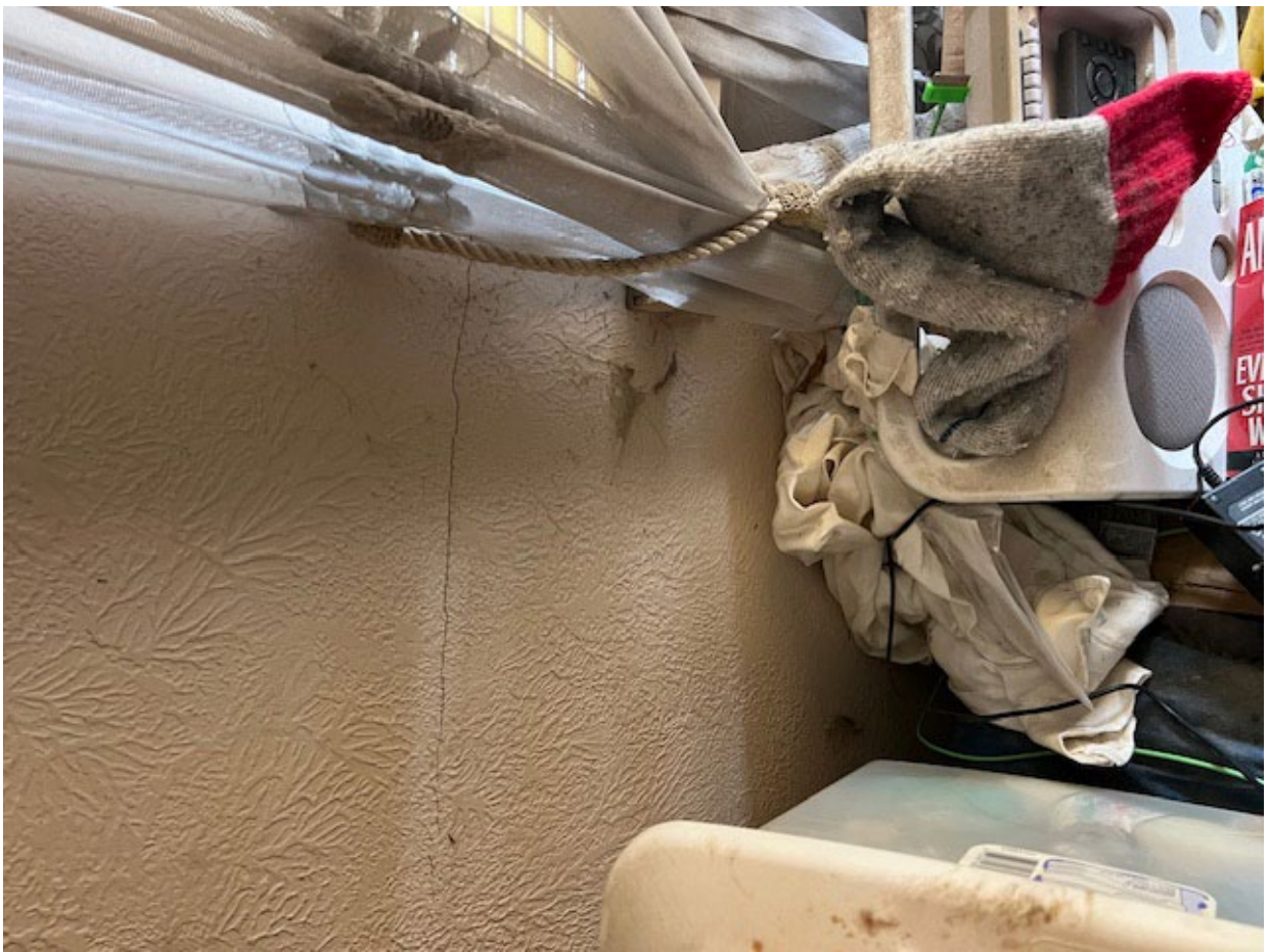
Settling under east bedroom window
