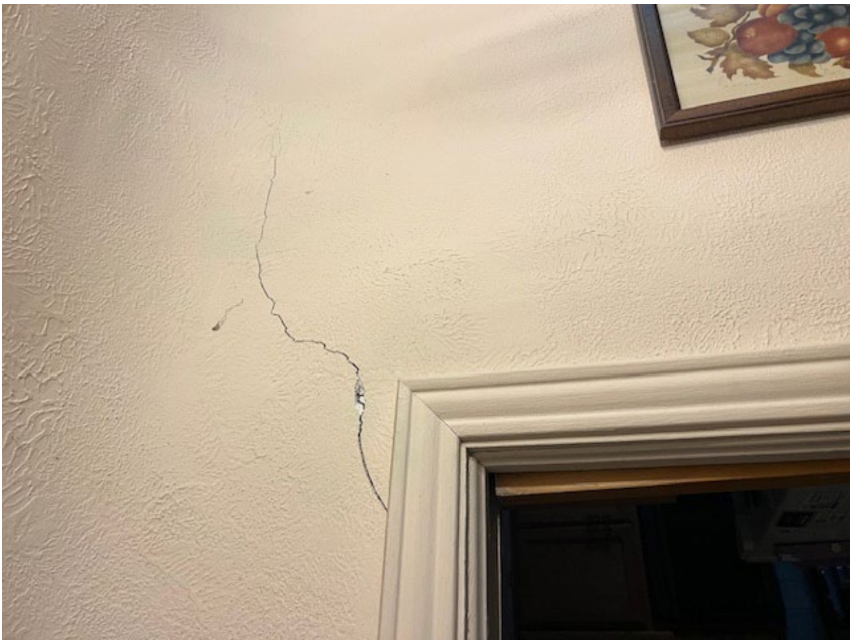
Signs of settling on east side of arch in living room area
