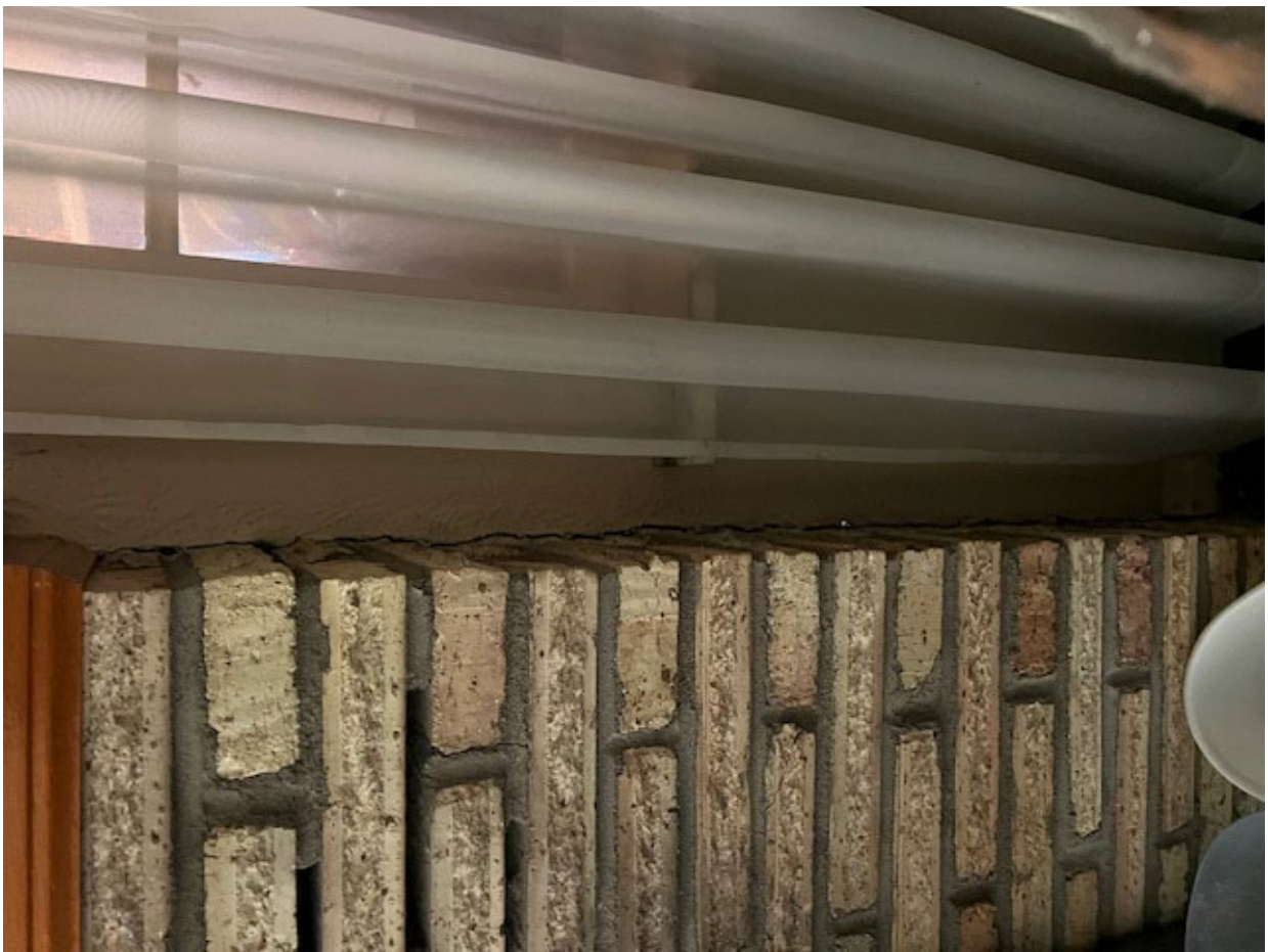
Settling in the wall over the arch (on west side of arch) from the bathroom to living room
