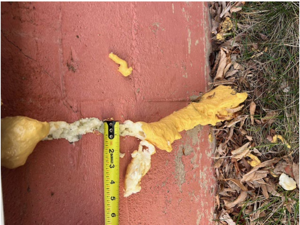
West Side of Chimney where the chimney has separated from the house there is a large “patch” of caulk and metal for drainage issues
